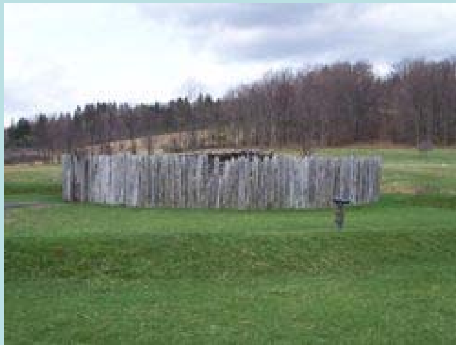
Fort Necessity near Farmington, PA (Modern Reconstruction)
